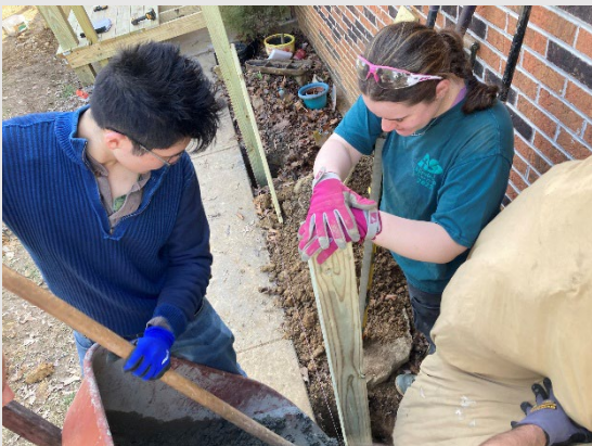
Me and my team working on setting the foundation of a wheelchair ramp during my time at Bethlehem Farm.
